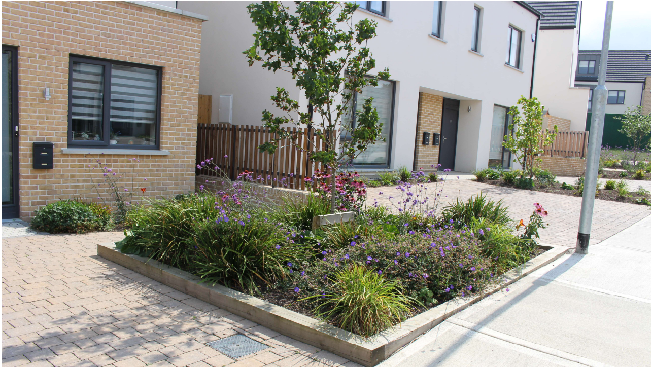
Figure 25: Typical planting bed timber edging at Scholarstown Wood by DFLA.
