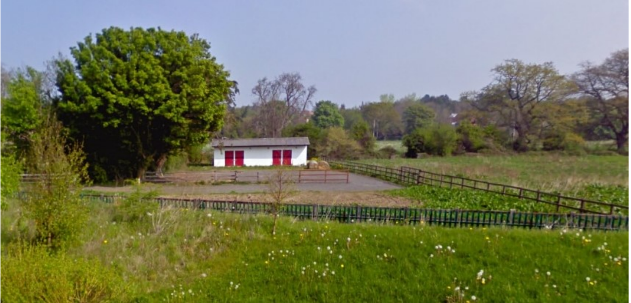
Figure 7: Western boundary: existing fence around private property (blue zone in Figure 2).
