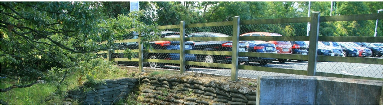
Figure 8: The boundary separating the site from the Carrickmines Luas Park and ride car park (Yellow zone in Figure 2) consists of a timber and chain-link fence.
