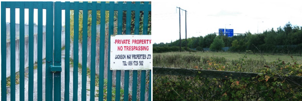
Figure 6: Southern boundary: gate to underpass (left), view to the M50 from over the existing south barrier (right).
